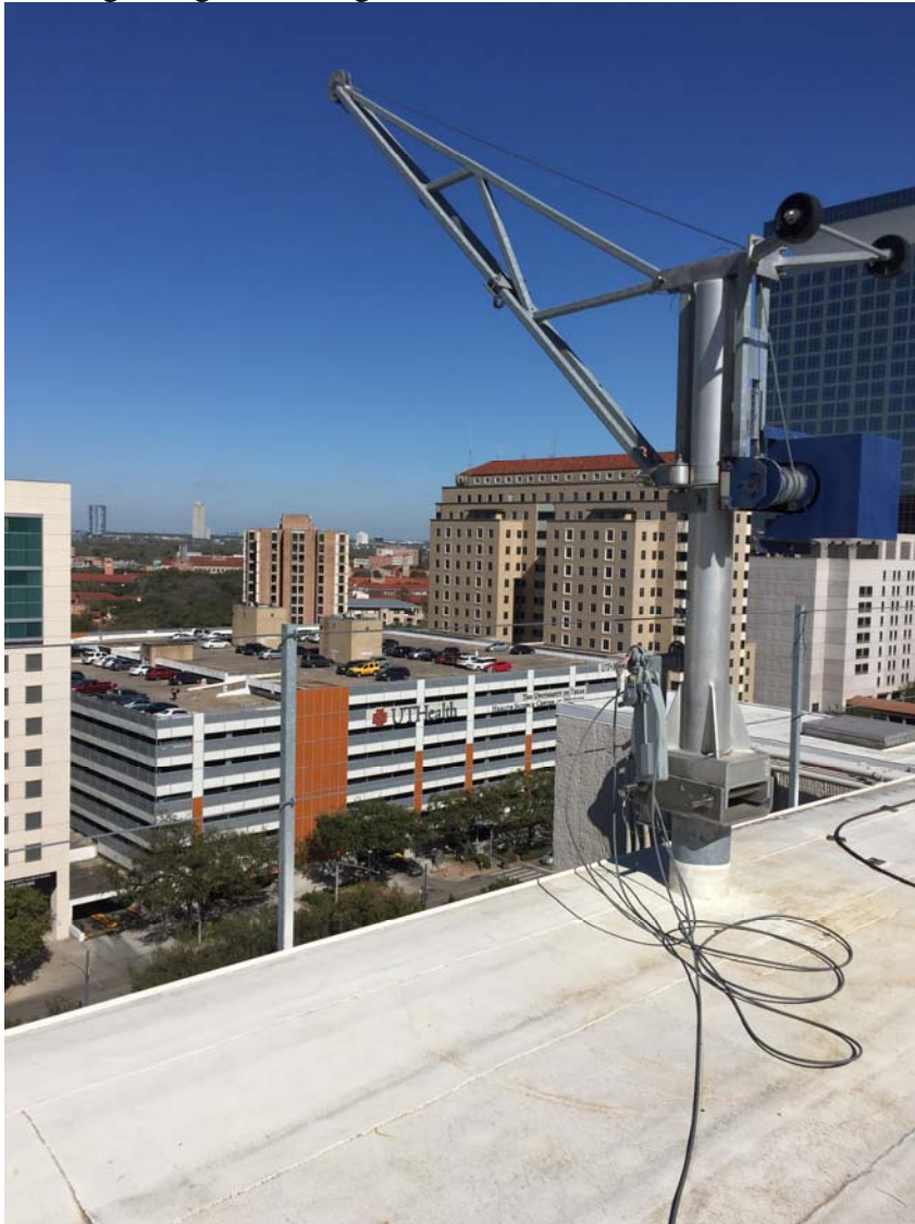
Existing swing arm on high roof:
